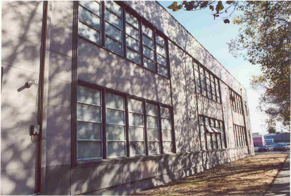
Figure 3: South Elevation of Main Classroom Building (window wall)
