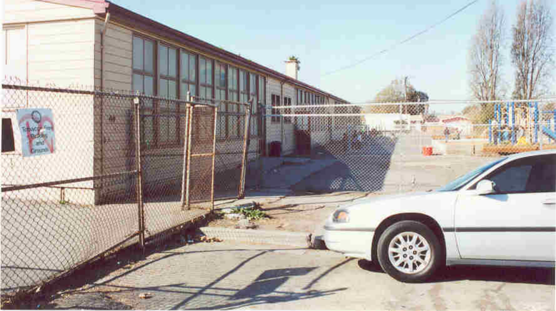
Figure 7: North Elevation of Kindergarten (Window Wall)
