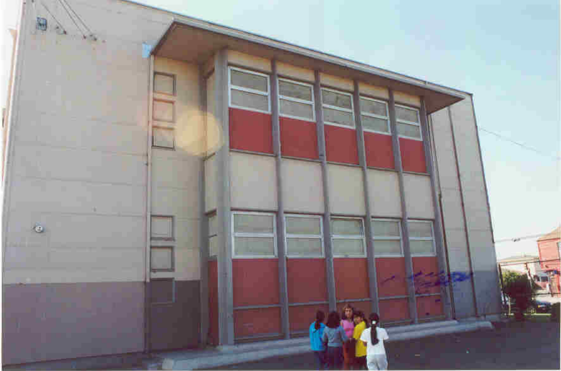
Figure 5 North of Main Classroom Building
