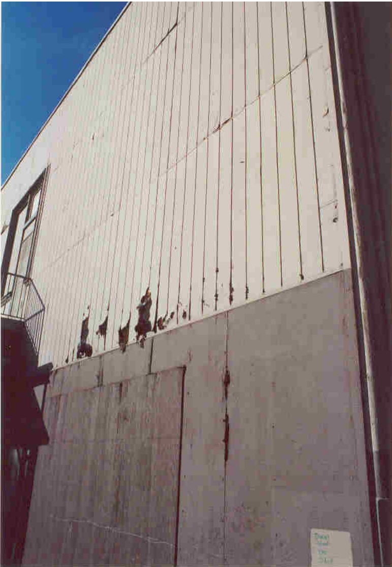
Figure 4: East Elevation of Main Classroom Building (siding decay)
